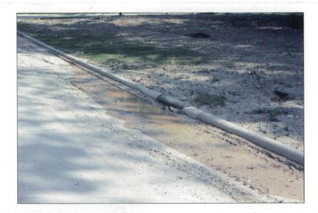
Surface flow inlet protection is necessary where these inlets drain areas of bare and unprotected soil surface(s). Geotextile wrapped around the frame and secured properly allows water to filter through. A structurally sound unit is needed to withstand the weight of sediment-laden water.
