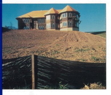
Silt fence can be an effective sediment control practice on individual lots during the house construction phase. They keep sediment from getting into the streets and street inlets, and from damaging neighboring lots.
