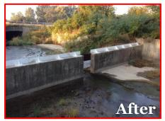
provide an additional 11 million gallons of storage at the West Point basin, and more importantly, reduce the base flood elevation six inches in the Pitts/Gina area.
