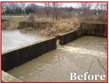
Modifications were made to the West Point weir to take better advantage of the available storage in the 22-acre West Point detention basin. The primary orifice was reduced by half and the height of the weir was increased by 18 inches. Reducing the orifice size reduces the flows permitted to continue downstream and raising the height increases the amount of water that can be stored and released later. Completing this first step alone in our multi-step plan will
