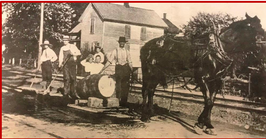
A work crew spreads oil on Center Ridge Road in Ridgeville Township in 1915 to keep down the dust.
