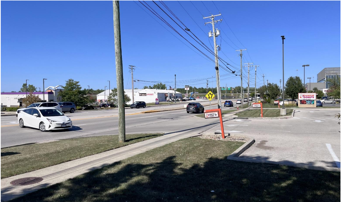
Figure 8 - Vehicle Making U-Turn from Westbound Lorain Rd at Dunkin Donuts Drive
