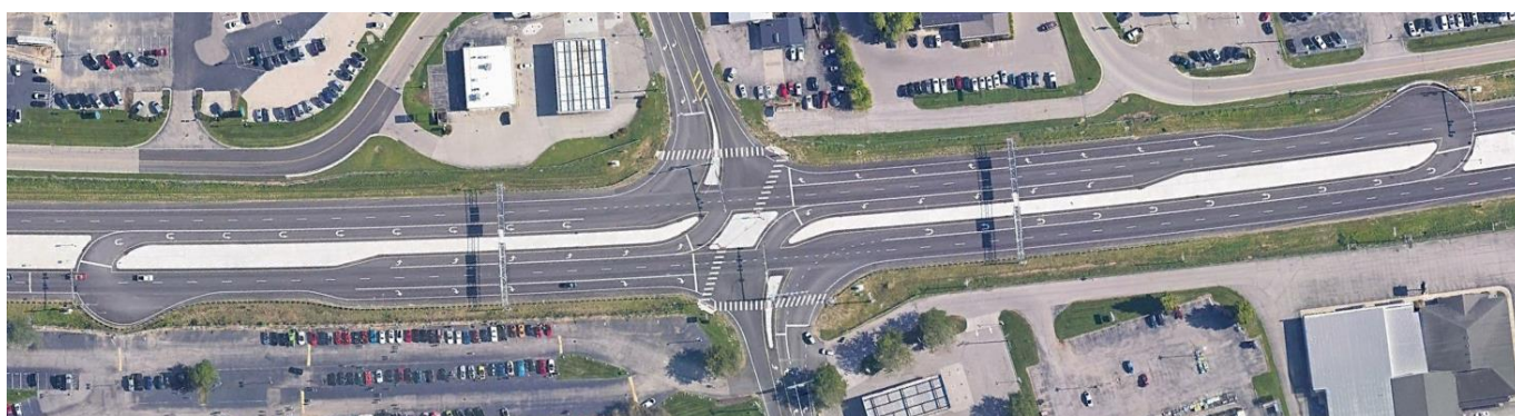
Figure 23 - Example of an RCUT Intersection: US 35 at S Orchard Ln, Beavercreek Township OH
