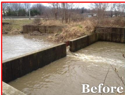
Modifications were made to the West Point weir to take better advantage of the available storage in the 22-acre West Point detention basin. The primary orifice was reduced by half and the height of the weir was increased by 18 inches. Reducing the orifice size reduces the flows permitted to continue downstream and raising the height increases the amount of water that can be stored and released later. Completing this first step alone in our multi-step plan will
